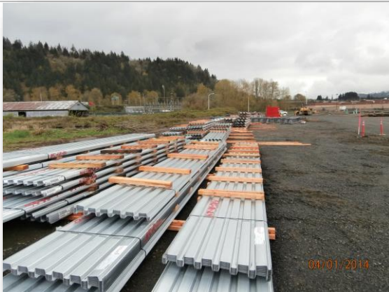
Stock piled metal deck
