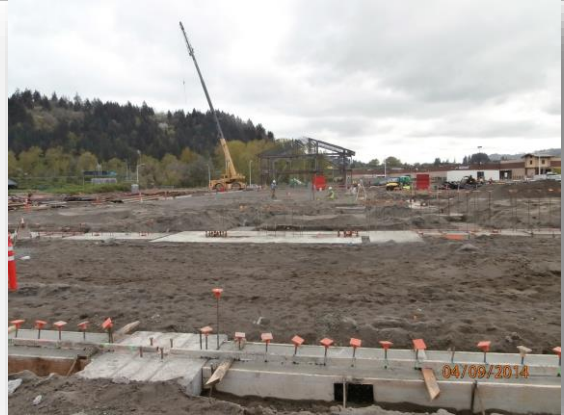
Ongoing foundation work
