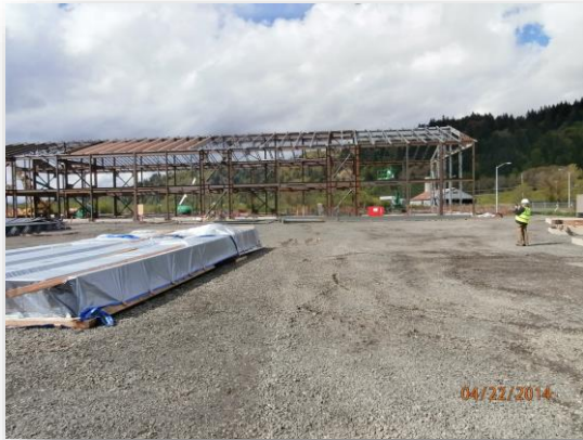
North Classroom Wing framing
