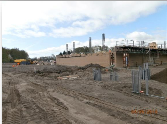
Main Gym wall construction
