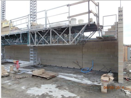
CMU installation at Main Gym
