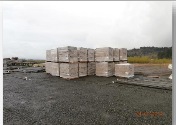
Stock piled concrete block
