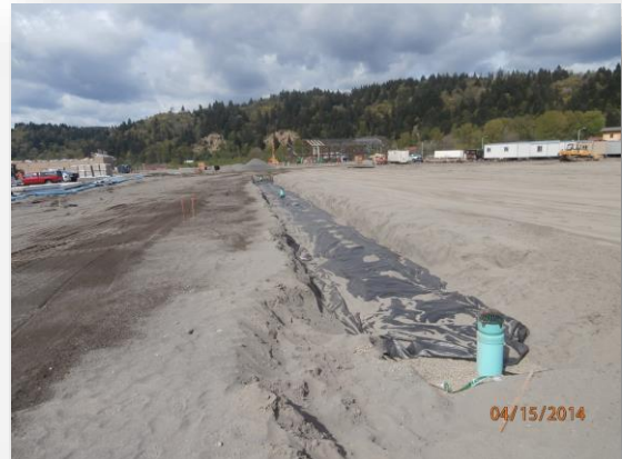
Infiltration swales at south parking lot
