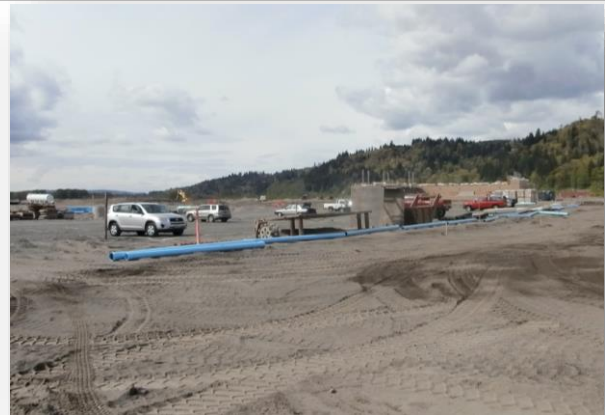
Storm sewer installation at south parking lot
