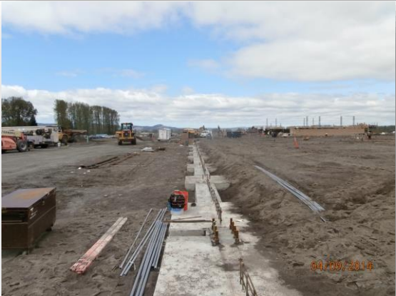
Ongoing foundation work
