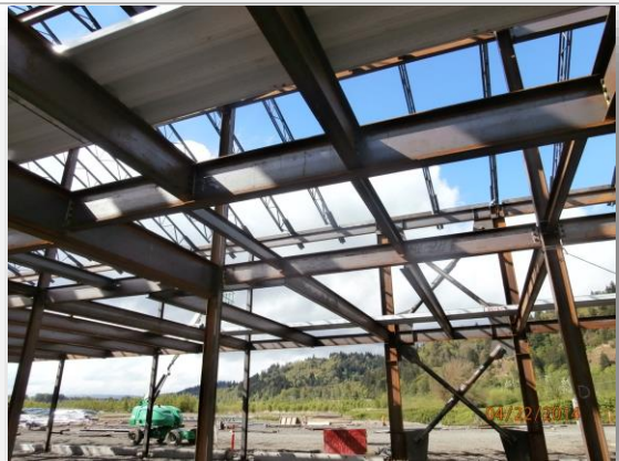
North Classroom Wing framing
