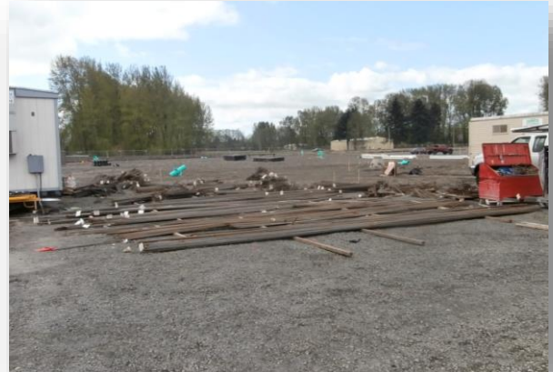
Stock piled rebar
