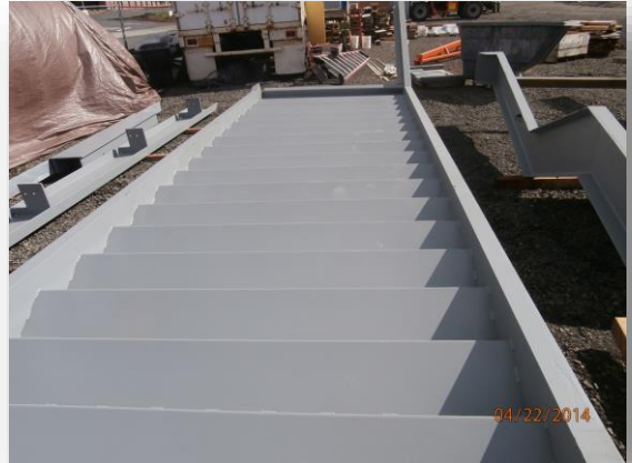
Fabricated stairs prior to installation
