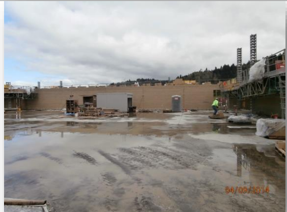
Main Gym slab and wall construction
