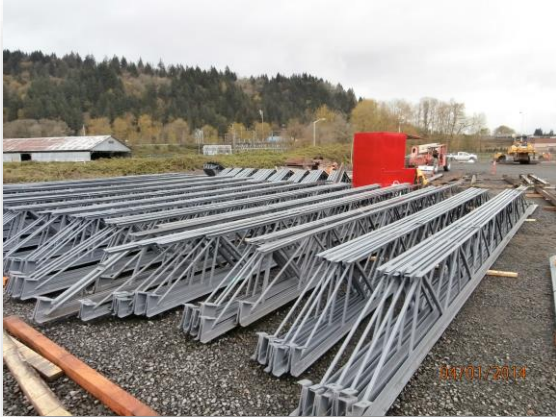
Stock piled roof trusses
