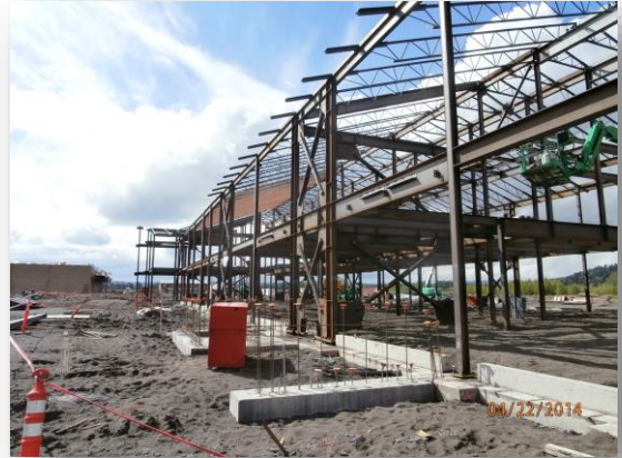
North Classroom Wing framing
