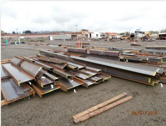
Stock piled structural steel
