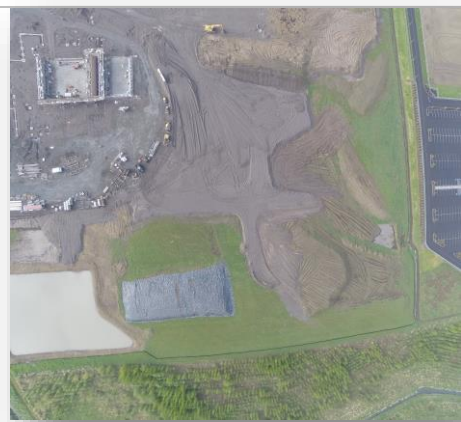
Aerial photo (NW corner/athletic fields)
