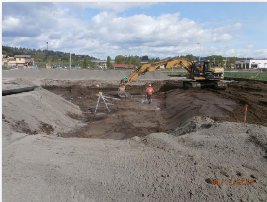
Rain Garden at SE corner of parking lot
