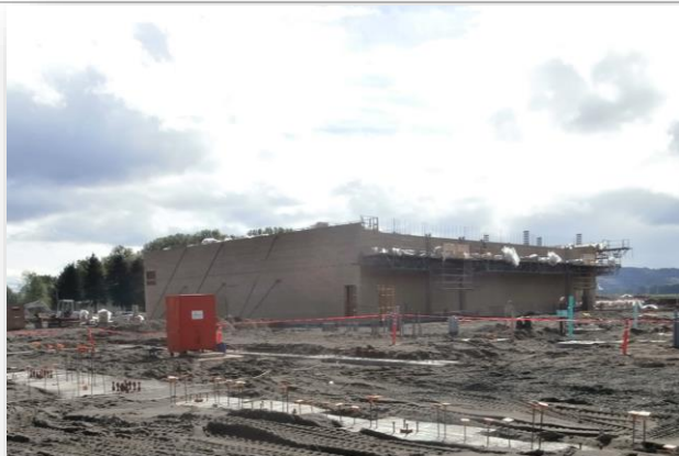
Main Gym wall construction
