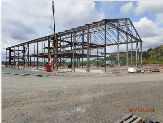
North Classroom Wing framing
